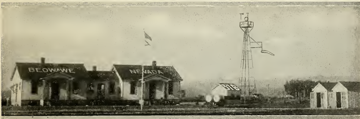
Airways keeper's quarters, teletype station, radio marker beacon and fuel storage tanks at an intermediate field
